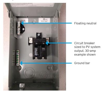
SDG&E will supply a circuit breaker sized to the PV system output as stated in the RMA request form, per NEC code calculations.
